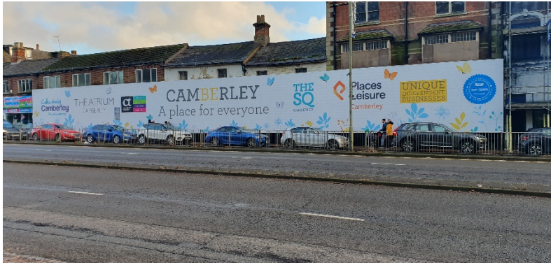
Hoarding Elevation looking southeast
