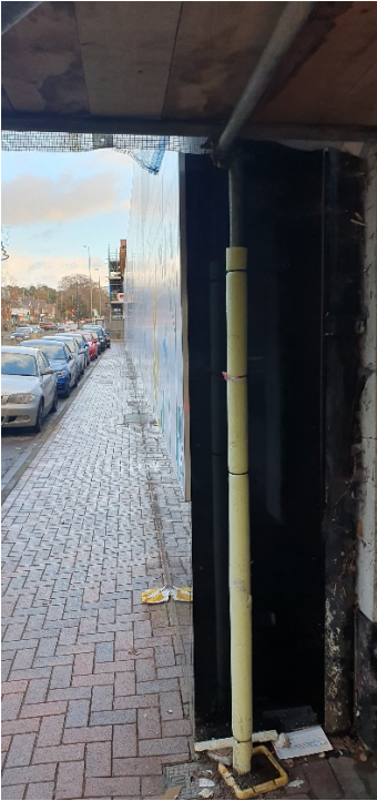
Hoarding side elevation looking northeast
