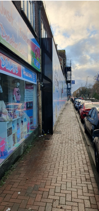
Hoarding side elevation looking southwest
